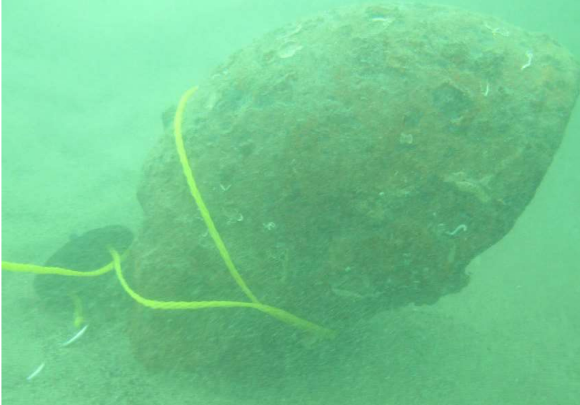
Photograph 15. Ocean outfall diffuser. Note sand covering outfall pipe.
