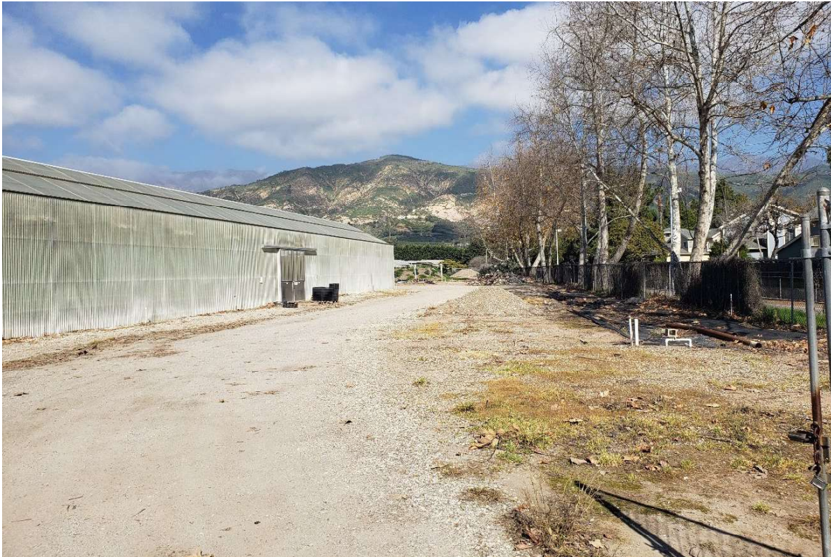
Figure 6 Injection Well Location 6, Facing Northeast
