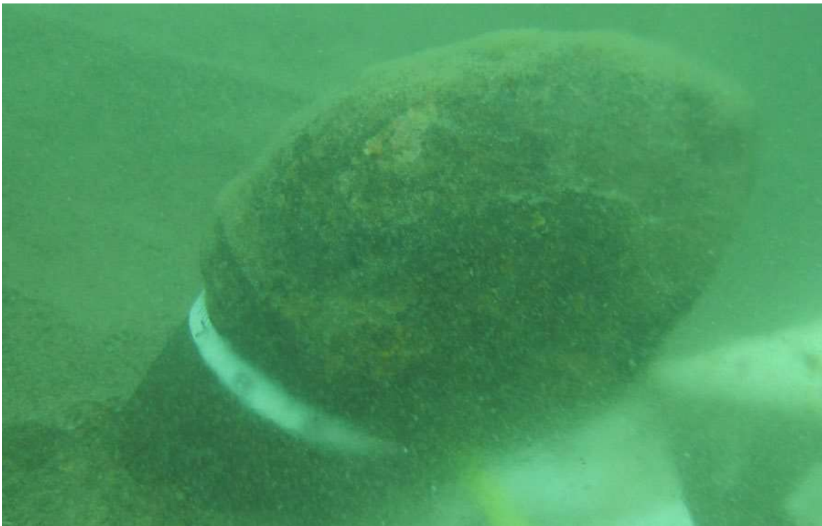
Photograph 18. Ocean outfall diffuser. Note diffuser actively discharging low saline water.
