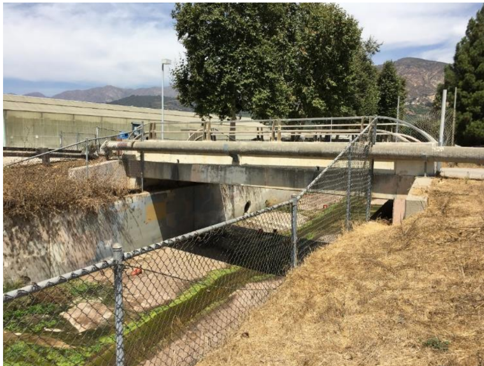
Figure 2-12. Existing Franklin Creek Pipe Bridge
