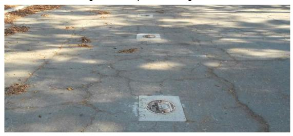
Figure 2-9: Example of Monitoring Wells
