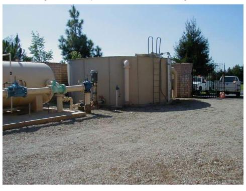
Figure 2-7: Example Well with Backwash Storage Tank
