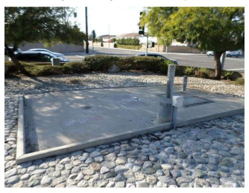
Figure 2-5: Underground Well Vault Example
