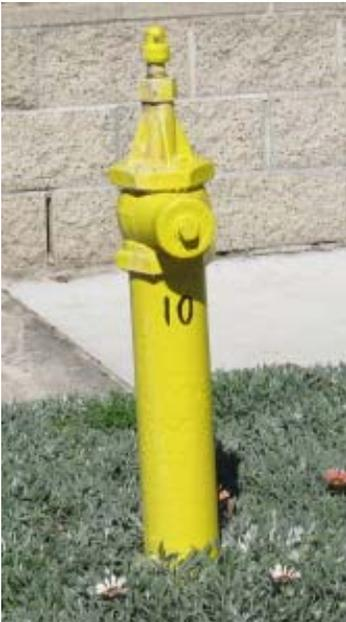
The fire hydrant pictured on the left is the old "wharf-style" hydrant with a 2 1/2" connection.
