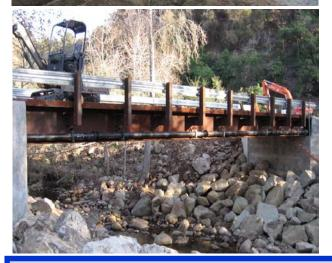
Restoration with cooperation from the Carpinteria Creek Watershed Coalition. A portion of the project involved removing the District's waterline out of the creek bed and fastening it to a newly installed bridge to keep the line protected.
