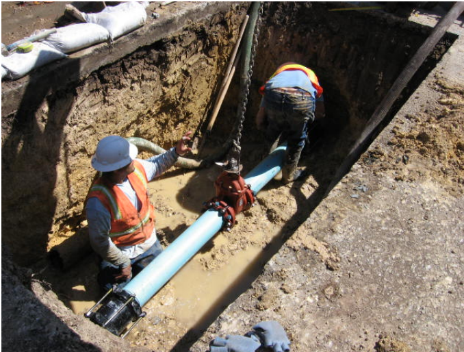
Pictured above are Carpinteria Valley Water District field staff installing two new valves in the Concha Loma area.
