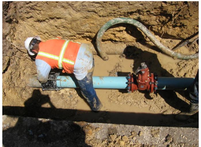
Pictured above are Carpinteria Valley Water District field staff installing two new valves in the Concha Loma area.
