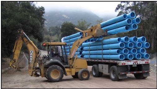
Pictured at left, is the offloading of some of the 12" PVC pipe that will make up the approximately 3000 feet of pipeline for Phase II of the CZ Main Extension Project.
