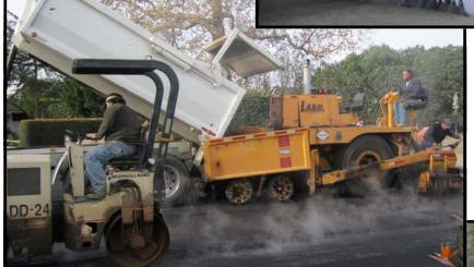
The photo to the left shows hot asphalt material being dumped into the asphalt spreading machine. The machine evenly disperses the asphalt and can adjust the thickness. The machine in the foreground is the rolling compactor.
