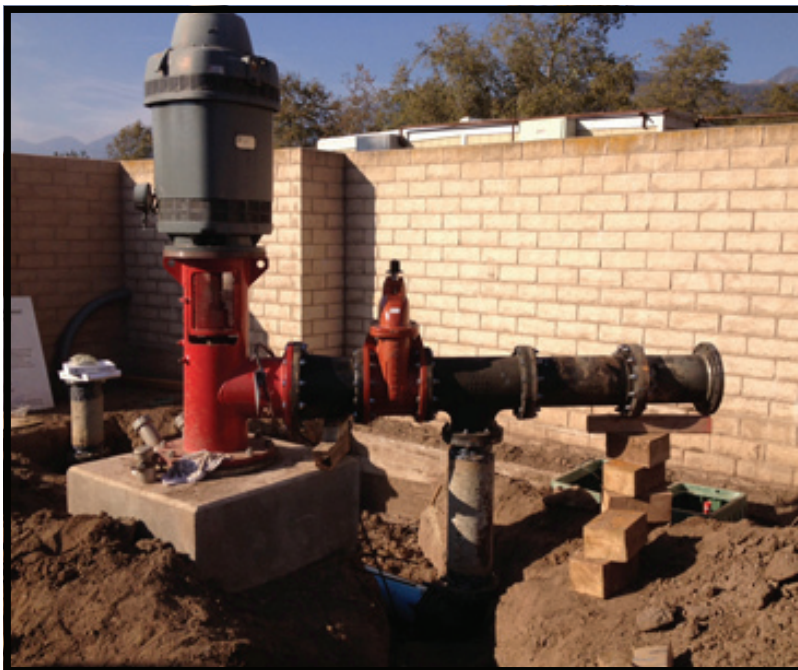
Pictured is the initial portion of the El Carro Well piping system to the on-site treatment plant.
