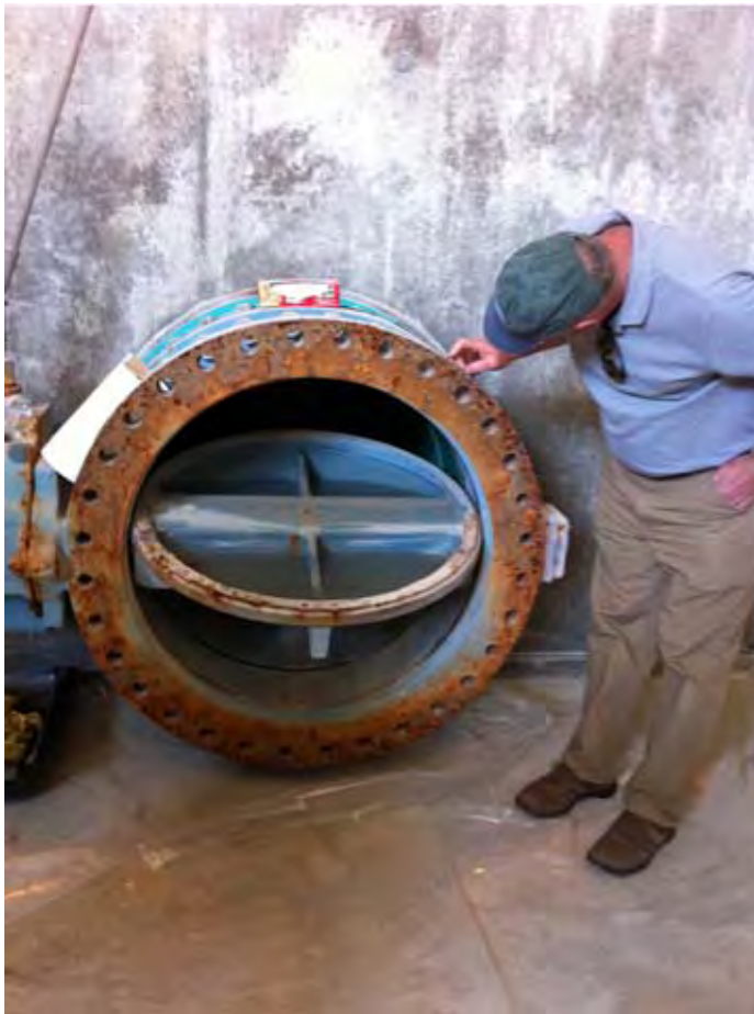
Pictured left, Director Matt Roberts inspects a valve corroded with rust which can also be seen in the picture on the right.
