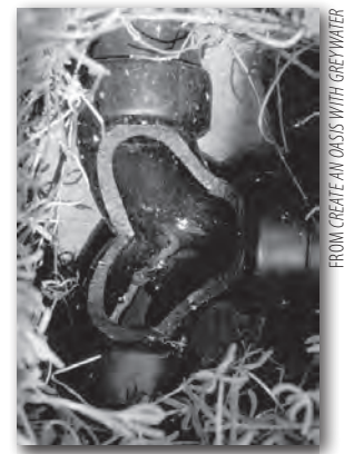
Cutaway view of flow-splitter; a fitting that is largely self-cleaning with no filtration.
