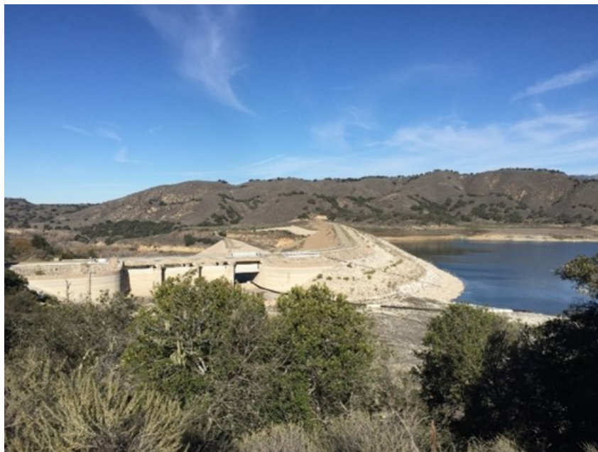
Figure 12: Photo – Bradbury Dam, Lake Cachuma, Santa Barbara County (December 2018)
