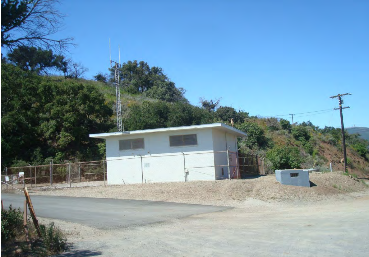
Photograph 7. View of the Rincon Vent Station; facing west.
