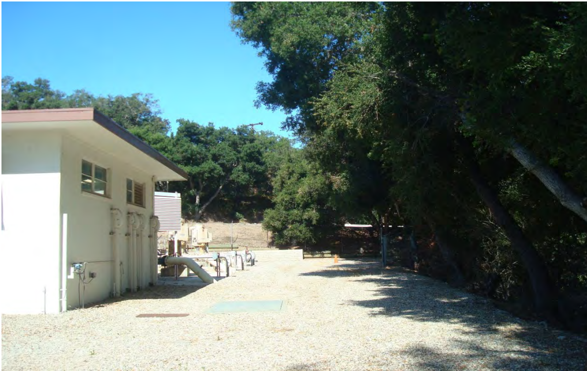
Photograph 6. Back view of the Rincon Pumping Plant and Coyote Creek to the right; facing west.
