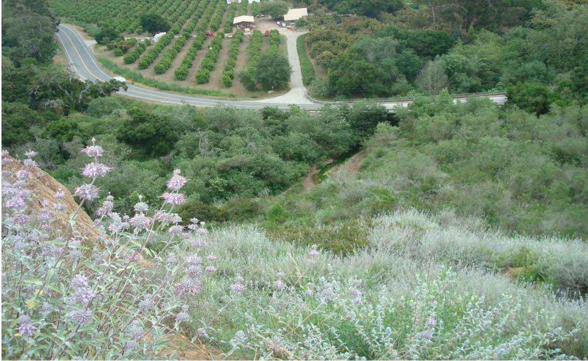
Photograph 3. Overview of Rincon Creek where HDD activities are proposed; view facing southeast.
