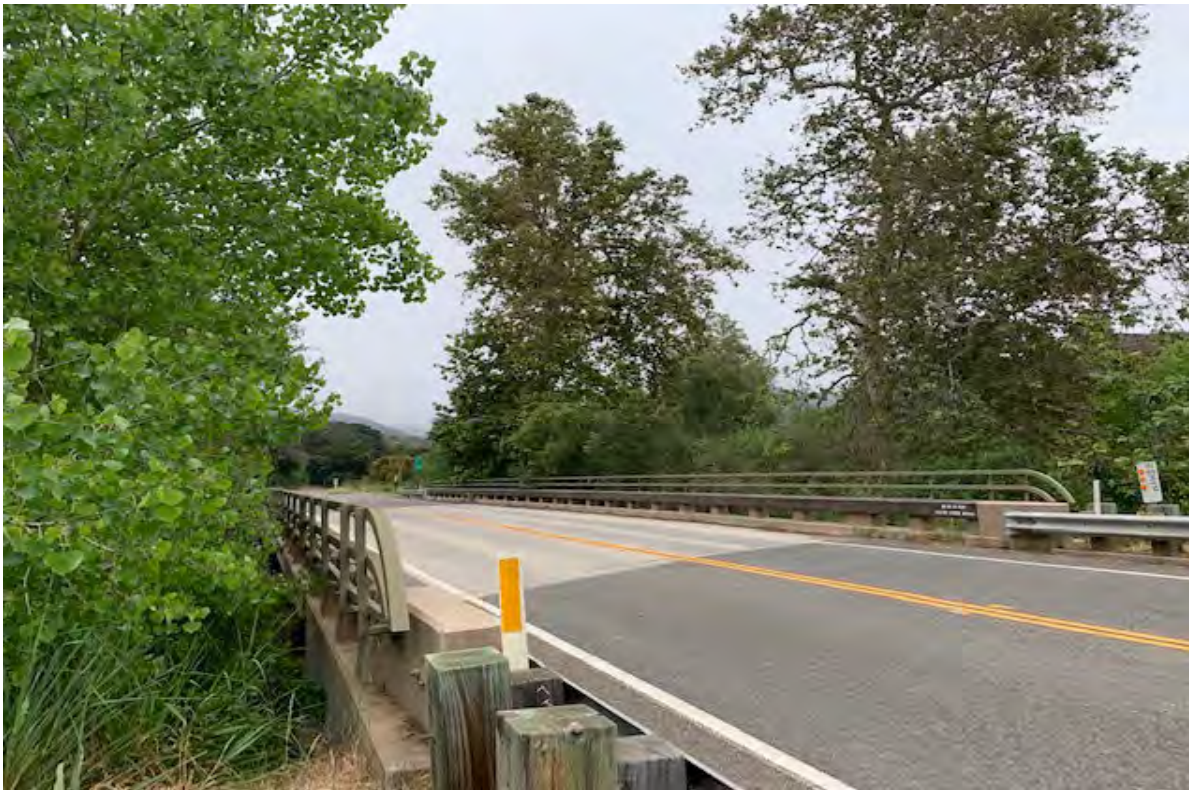
Photograph 4. View of Rincon Road crossing over Rincon Creek; facing southwest.
