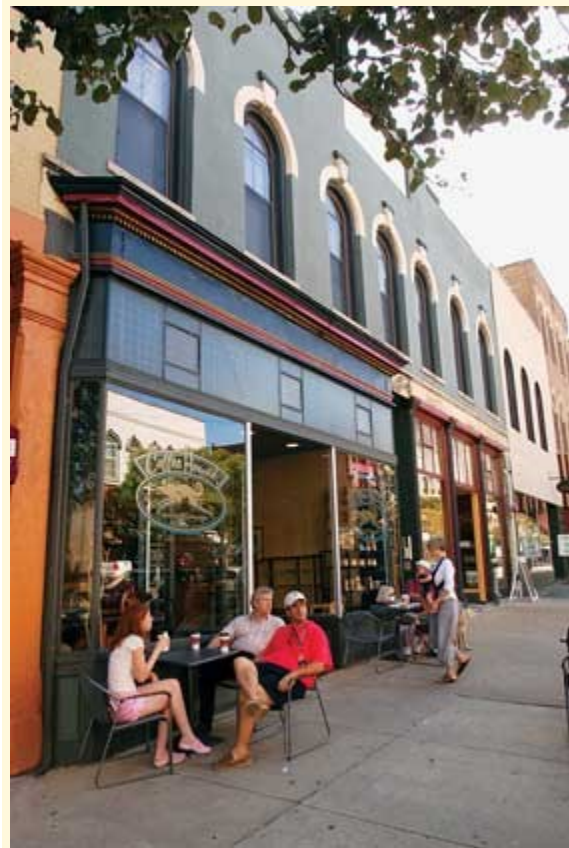
Figure 1 - Sidewalk café located near building to allow safe pedestrian access.
