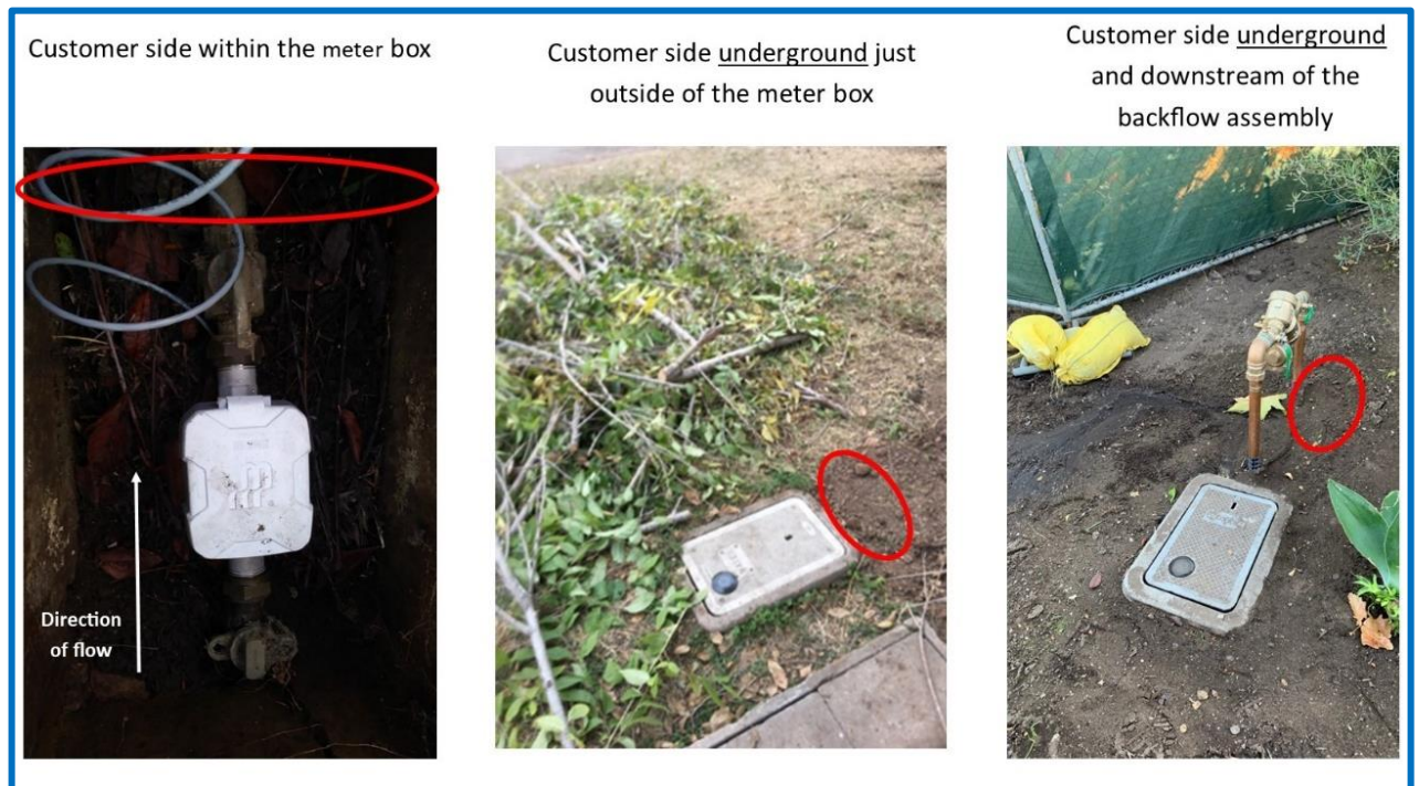
Figure 1. Options for Testing the Customer's Pipe Material
