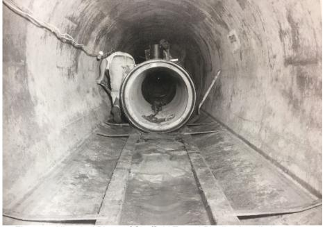
Figure 4. Historical Photo of Sheffield Tunnel Pipeline installation
