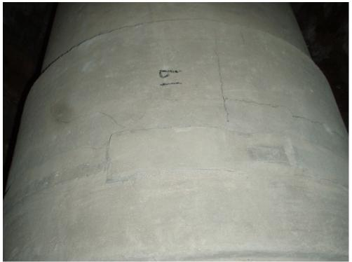
Figure 1. Centrifugal Concrete Pipe Joint Within Sheffield Tunnel Showing Minor Cracking
